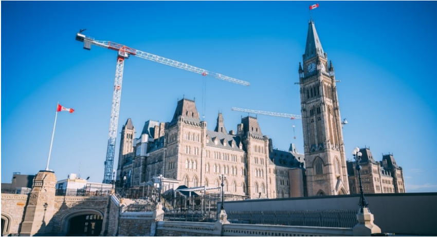
Centre Block under construction
